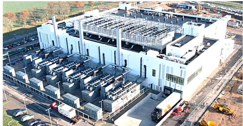
Data centers are industrial facilities in every way
