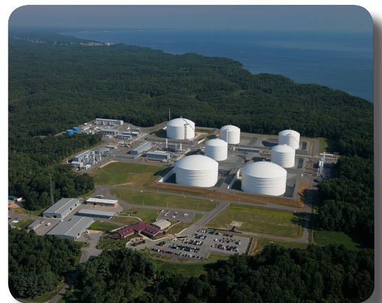
Aerial view of LNG Facility in Cove Point (Photo Credit: LNG World News)
